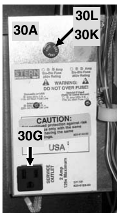
Enlarged Inside Cabinet View of Items 30: Power Box (30A), Service Outlet (30G), Fuse (30K) and Fuse Holder (30L).
